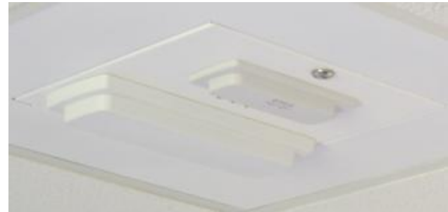
Rugged AP in ceiling enclosure
