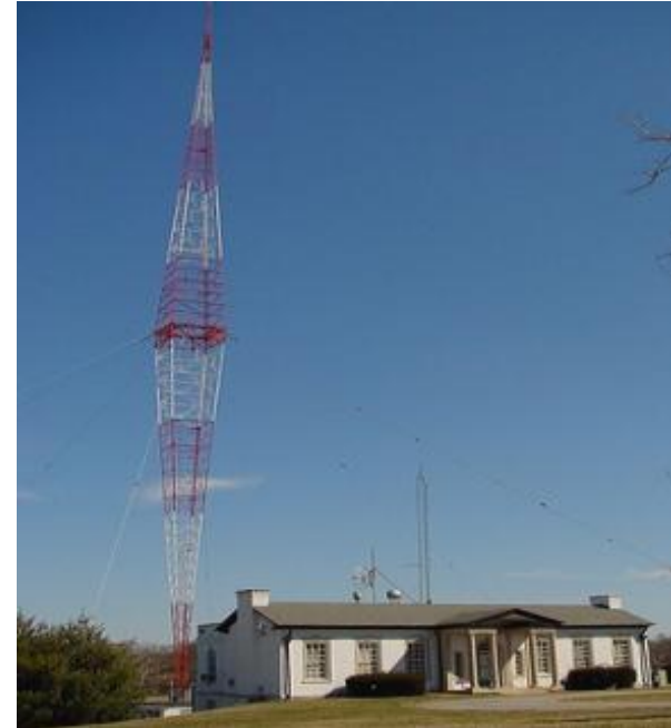
808 Ft Broadcast Monopole WSM 650 AM (erected in 1932)
